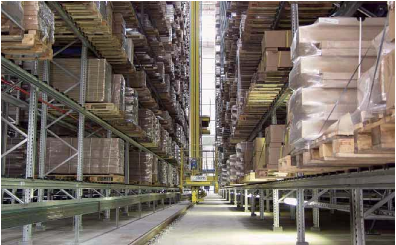
VKS 10 in high bay warehouses
