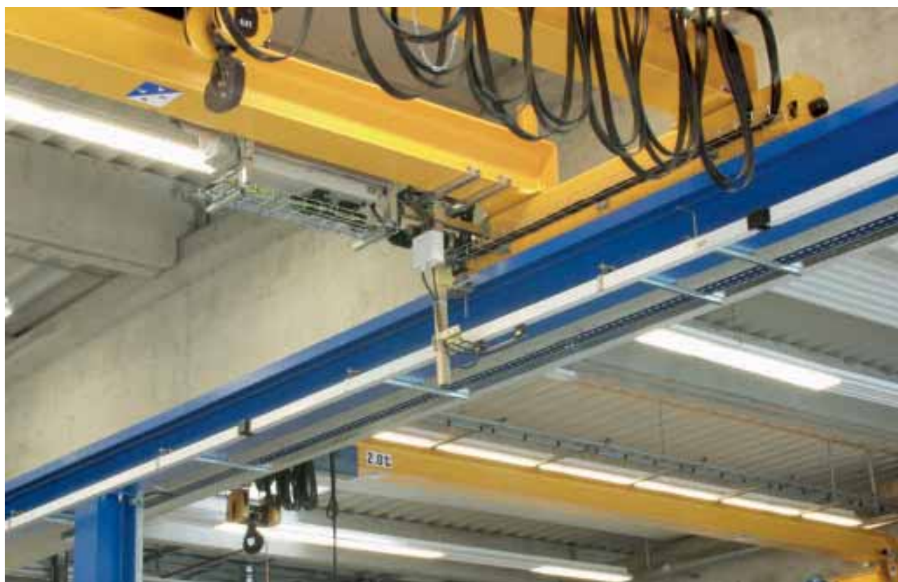
Crane installations at company Rheinmetall Landsysteme (Kiel)
